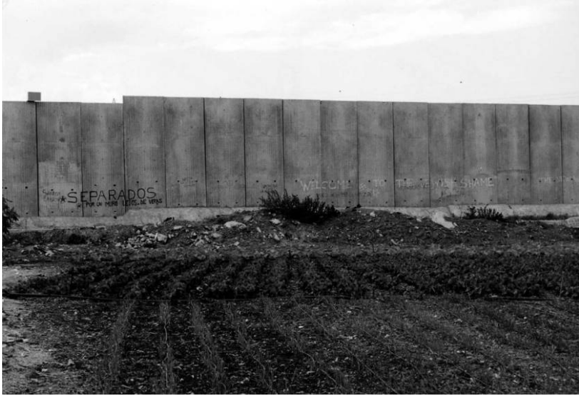
FIGURE 6. The wall, as seen from the Palestinian side, Qalqilya, West Bank. Photo by author.
