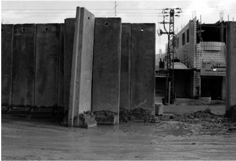
FIGURE 11. The wall under construction, al-Ram, East Jerusalem. Photo by author.
